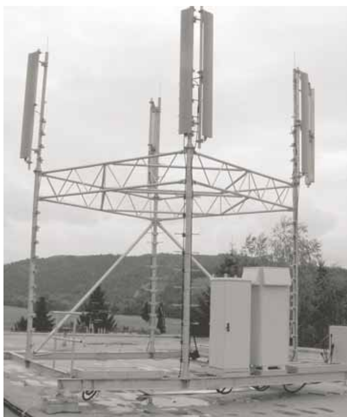
Base station GSM on the roof of the building – Nitrica
